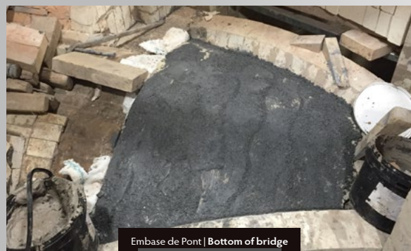
Embase de Pont | Bottom of bridge
