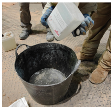
Empty the entire can of binder (B) into the container
