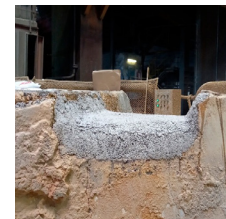
Repair example: Tundish spout
