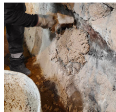
Application by trowel or vibrated casting
