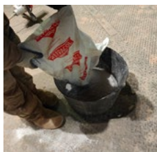
Pour the entire bag of Refravibre H800 Series (A) into a mixing tray
