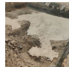
Repair example: Ingot mould bottom
